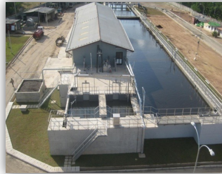
Ja Ela Ekala WWMP - (A2O) Capacity – 7,500 m 3 /day Population Coverage– 8,000(Domestic) + Industrial/ 73,500 PE
