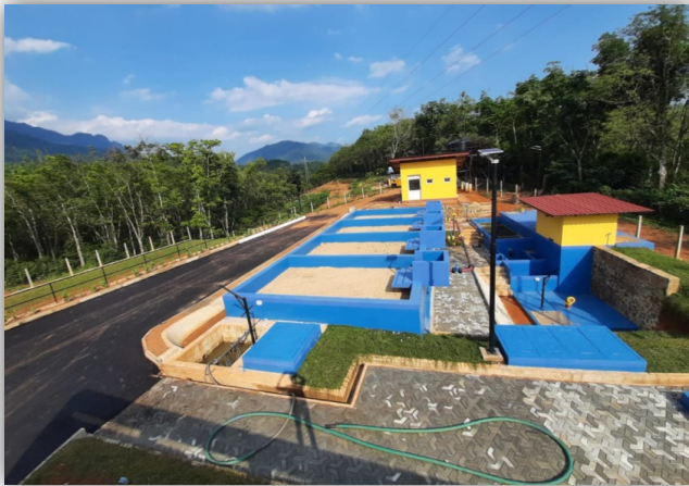
WELIGEPOLA FAECAL SLUDGE TREATMENT PLANT (25m 3 /day)
