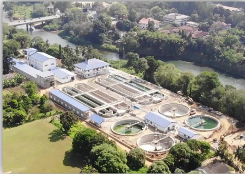
Kandy City WWMP- (Oxidation Ditch) Capacity – 14,000 m 3 /day Population Coverage– 55,000 (Domestic)
